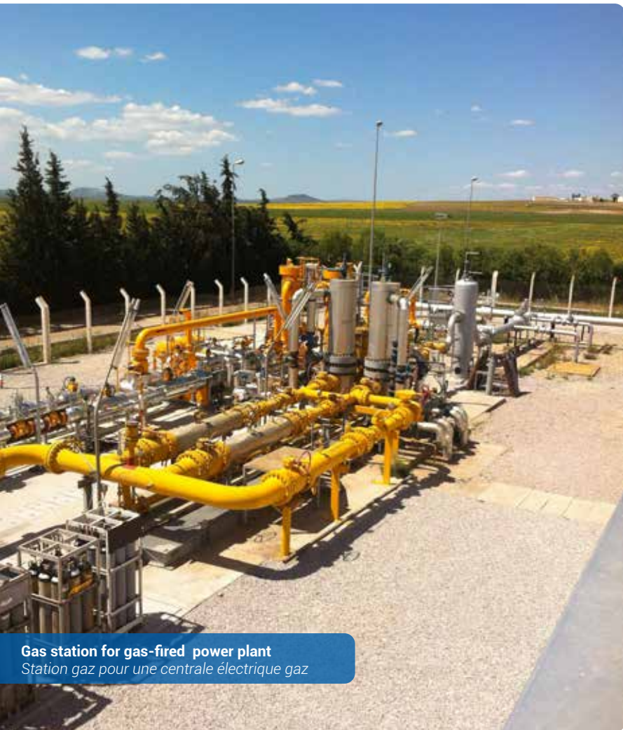
Fuel gas heating on gas station Réchauffage gaz sur station gaz
